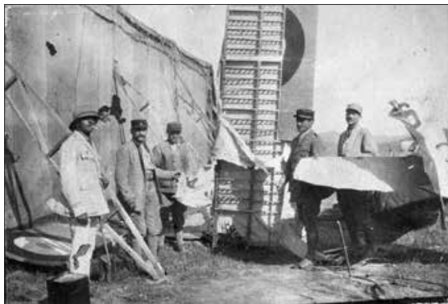
Views of the wreckage of Costes' first SPAD, S.1083, after recovery from the site of his crash landing on 8 July 1917. In addition to the fabric stripping off the top wing, note that the leading edge of the wing is missing as far back as the front spar. : David Méchin
